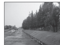
Wind barrier surrounding coal stockpile
