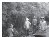
Dredging by employing local labors
