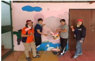
Paint the cafeteria and school
