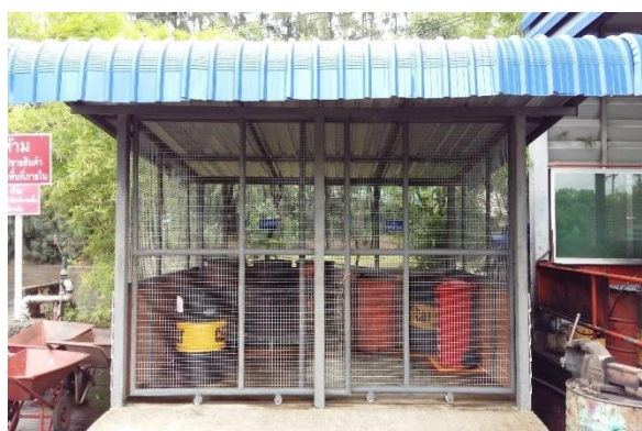
Storage Facility for Unused Materials
