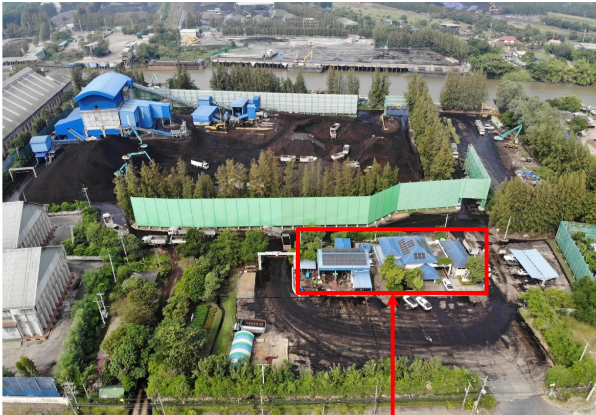
Picture shows the 24kW solar panel system installed on the rooftop of an office building at the Coal Distribution Center, Phra Nakhon Si Ayutthaya Province
